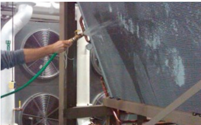
Easy to maintain – only water and a hose required to clean the coils.
